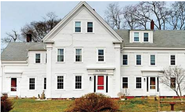
100 West Main St. An example of architecture of a varied massing, multiple roof lines, and contributes to the character of the area
