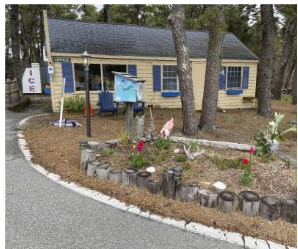
Office Building at Maurice's Campground
