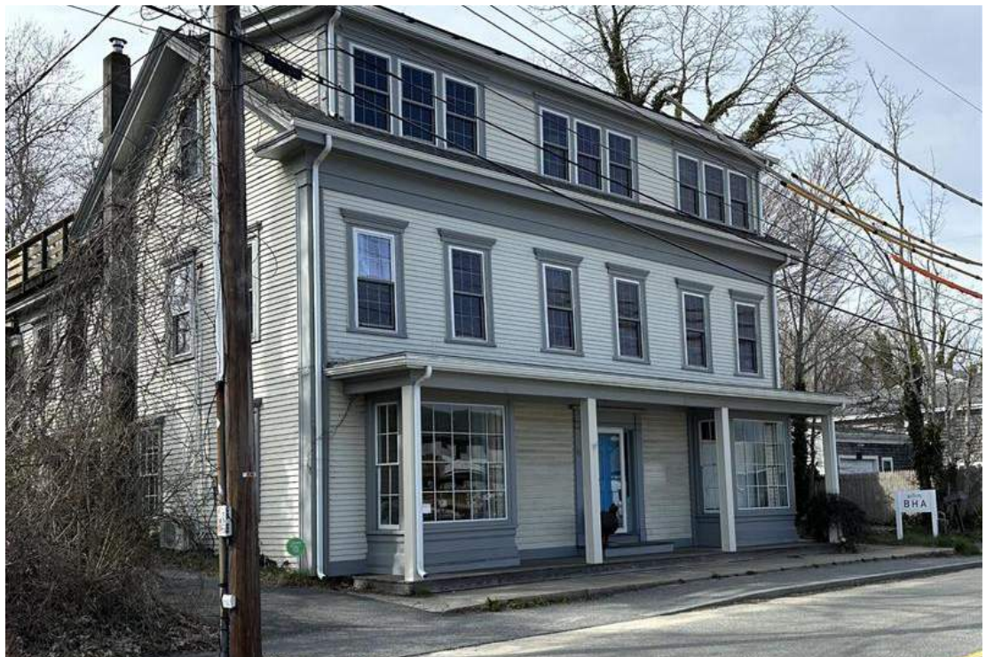
42 Commercial St in Wellfleet. This is an example of a 3 story building in Wellfleet.
