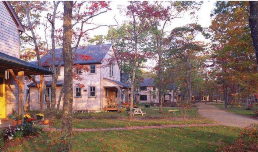
Island Cohousing on Martha's Vineyard. Front porches, variety of roof forms, natural materials.
