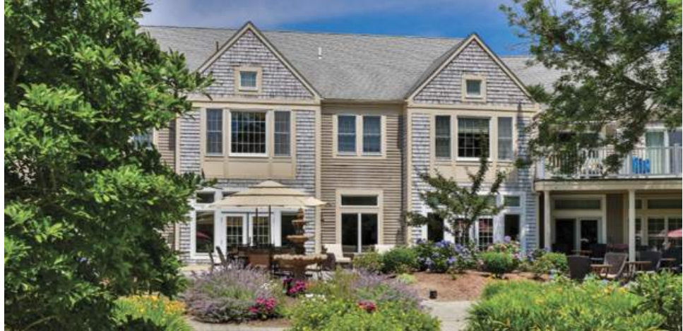
The Heatherwood in Yarmouth Port. An example of a building natural materials, facade changes to provide interest and variety.
