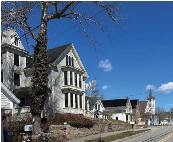
276 Main St. An example of architecture of a varied massing, with interesting details, and matches the character of the area
